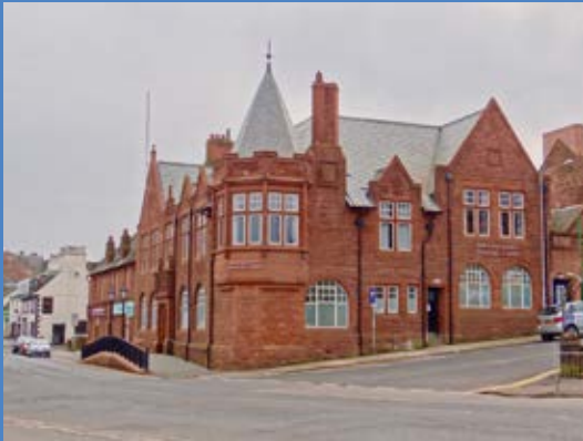
GOUROCK MUNICIPAL BUILDINGS
